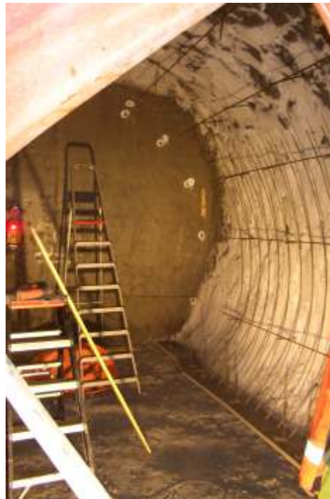
Excavated Cross Passage with exposed frozen walls
