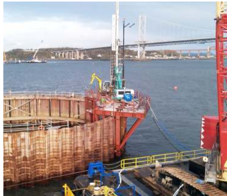
Forth Crossing bridge Scotland offshore Jet Grouting columns
