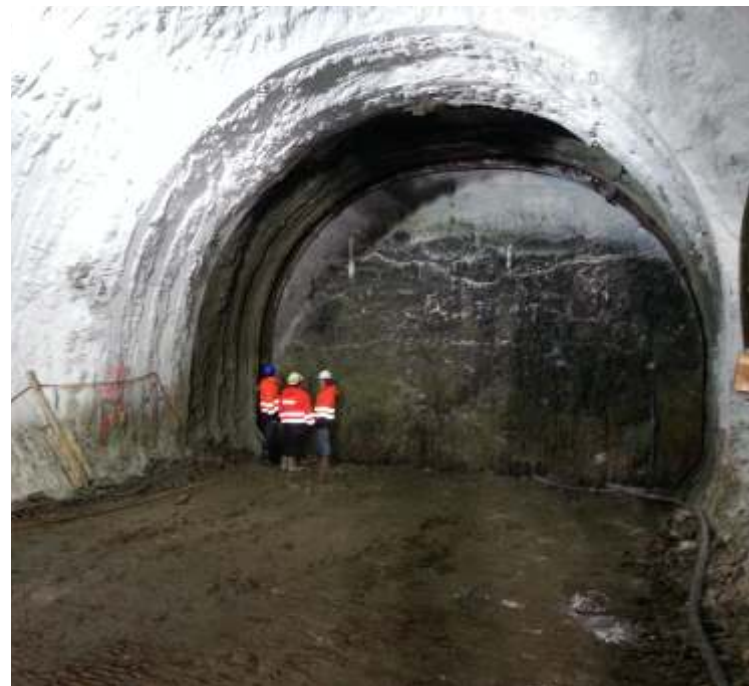
Metro Warsaw Poland C13 station Ground Freezing
