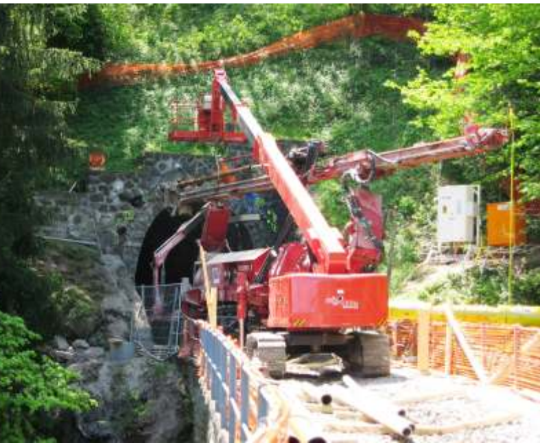
Tunnel Trositorrents Switzerland Forepoling
