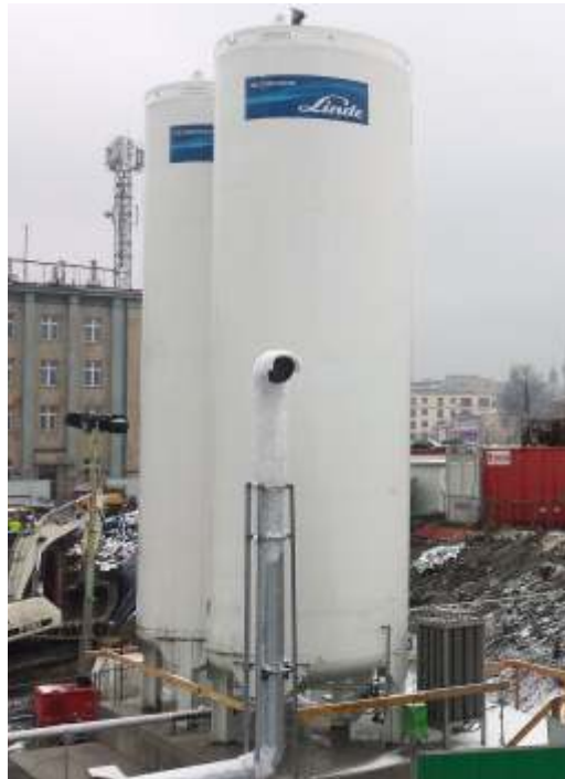
Liquid Nitrogen Tanks
