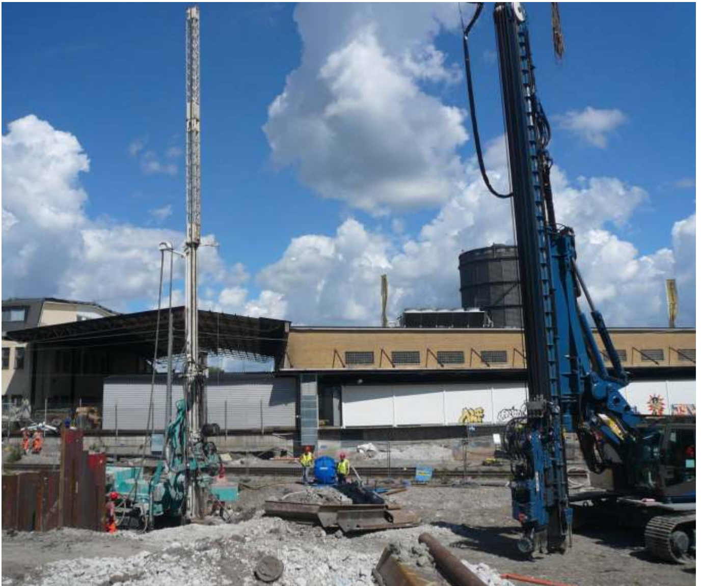
Casagrande C8 Super drill rig at work
