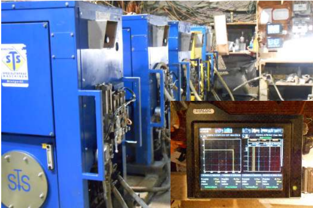
Grouting Plant with DIALOG GIN graphics on screen
