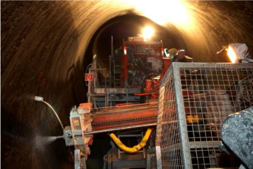
Drill rig inside the water discharge pipe
