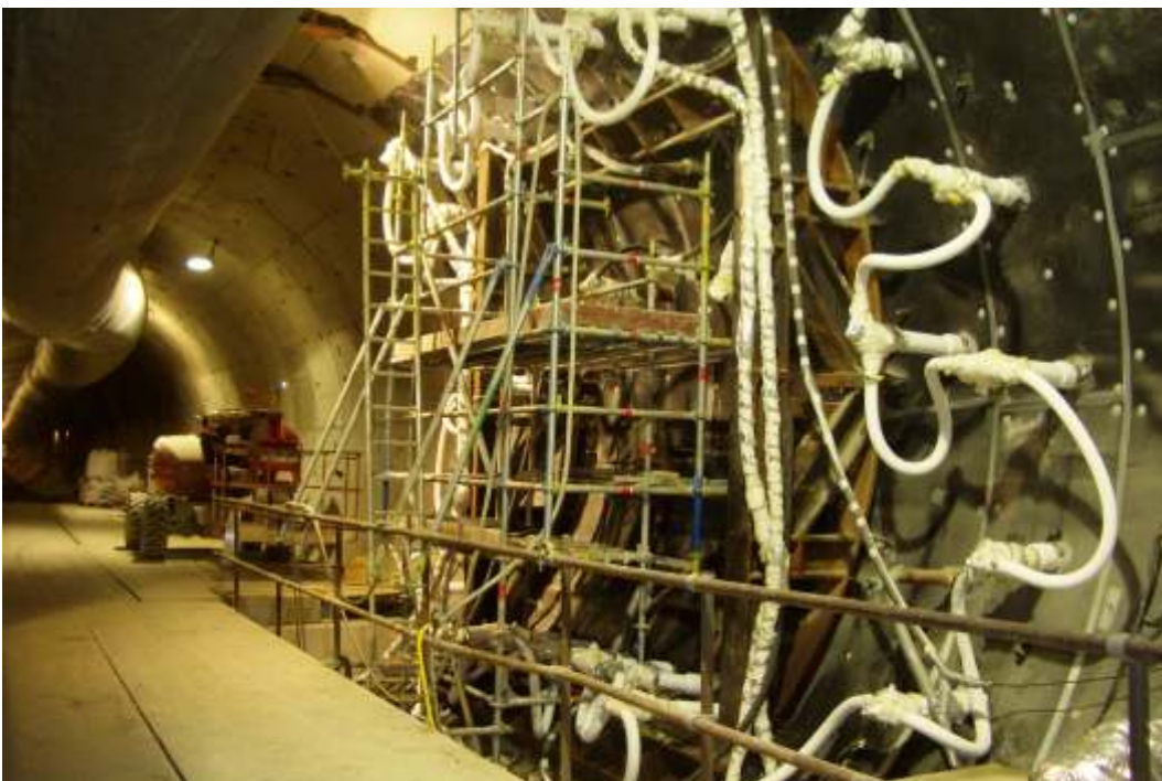
Brine distribution circuit and propping structure
