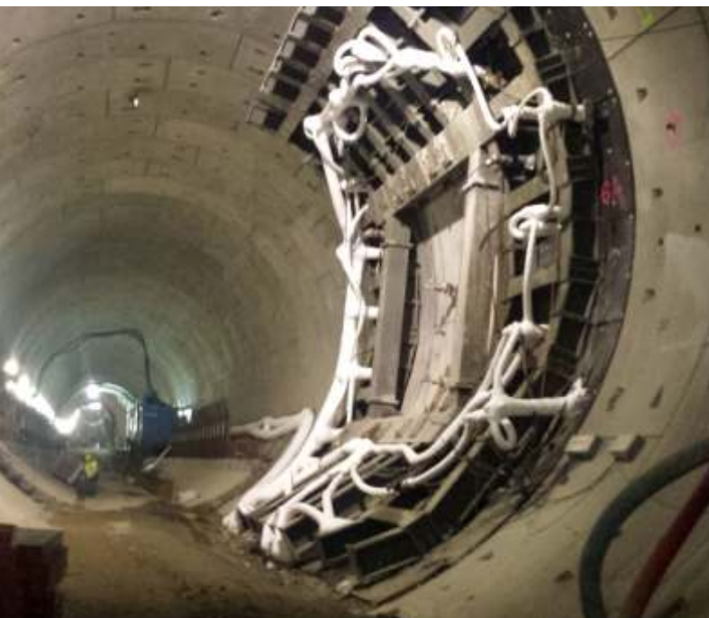
Slovacki tunnel Danzig Poland Ground Freezing
