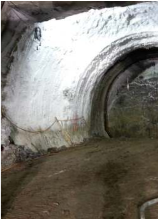
Frozen body seen from the tunnel
