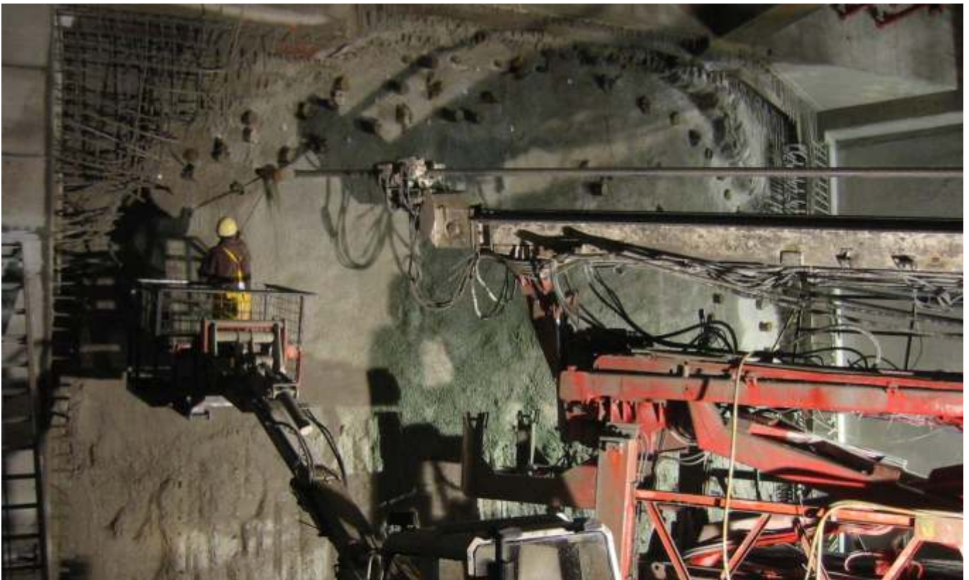
Placement of wooden plug
