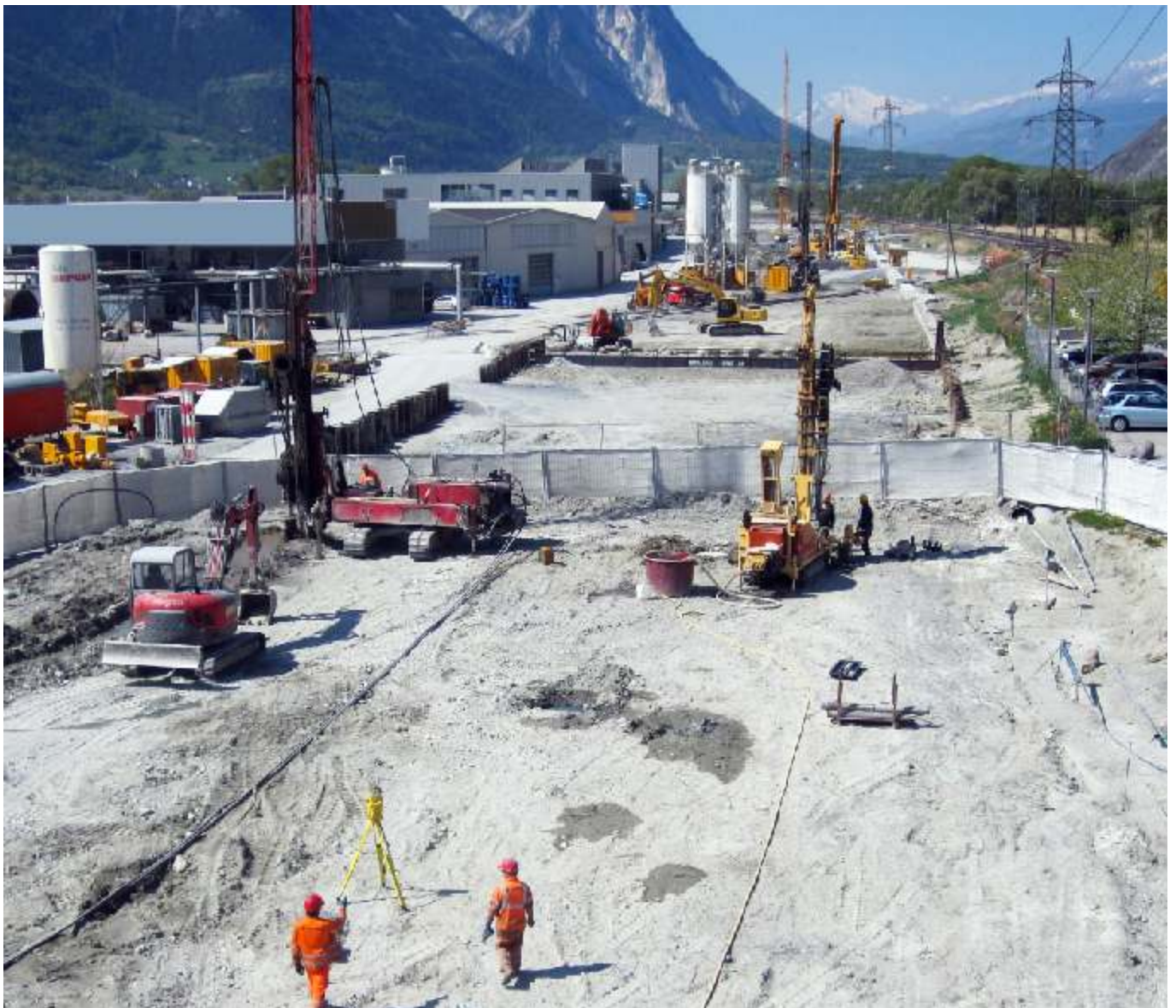
Drill rigs at work for the execution of the jet grouting slab
