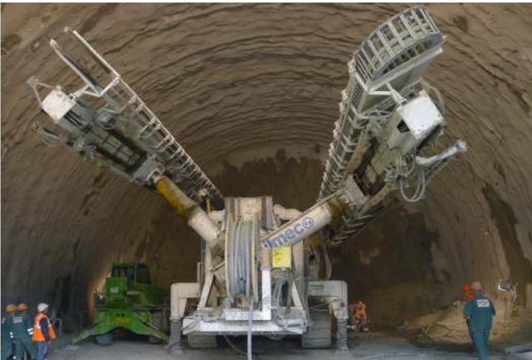
Double mast horizontal drill rig Soilmec ST120 at work
