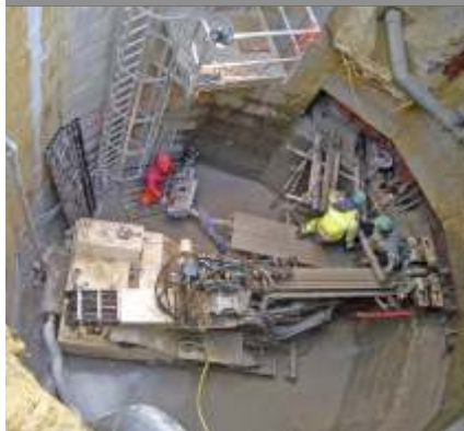
Compensation Grouting
