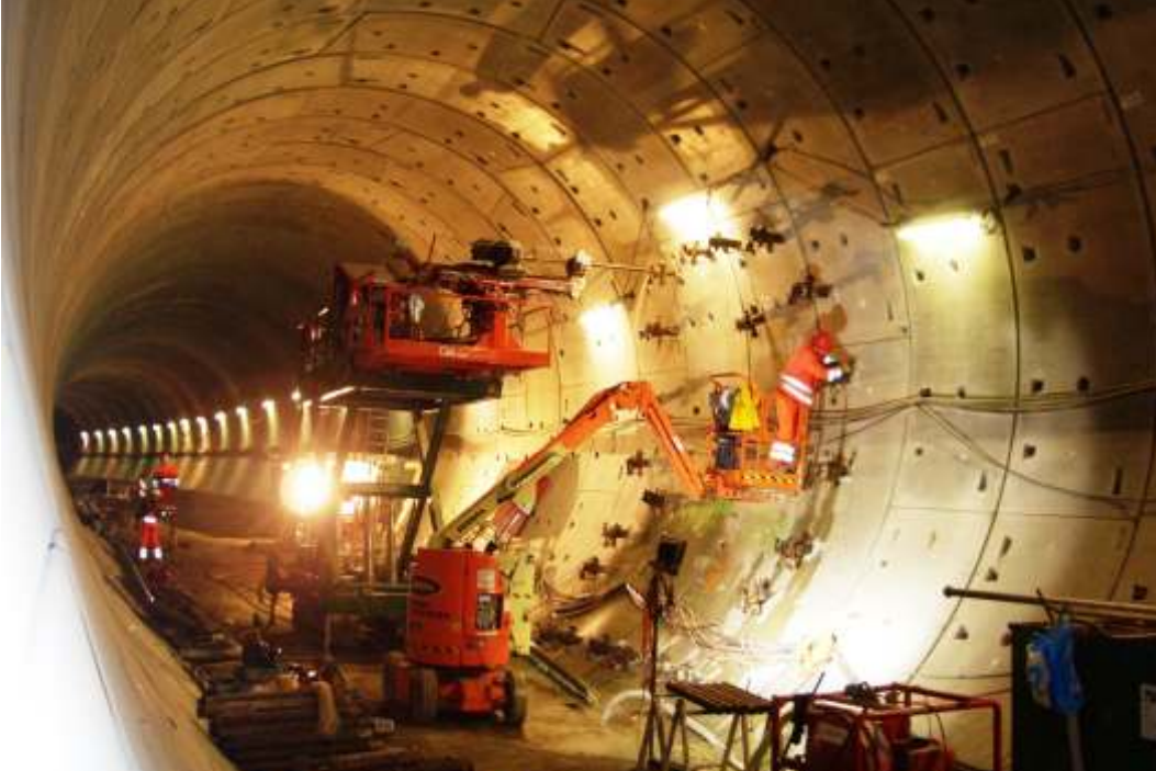
Platform mounted drill rig on a cross passage
